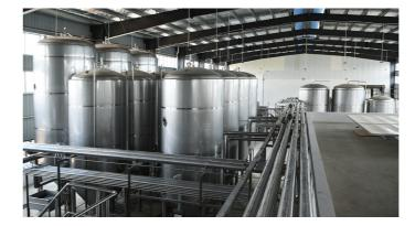
▶ The whole brewery is divided into several major modules by only connecting modules and related piping and electric wires on site, all the manufacturing and assembly, automation line connecting will be finished at factory before delivery to reduce the total construction cycle, minimize installation costs to achieve quick installation.
